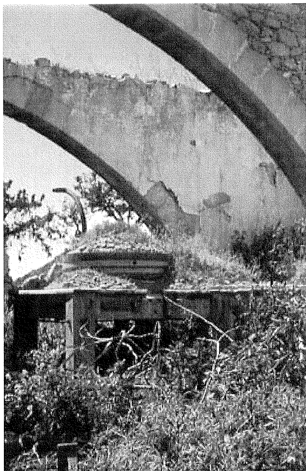
Fig. 8: Two pairs of millstones placed on a timber platform. Proto-industrial mill in Galinoporni, Karpasia, Famagusta district.
