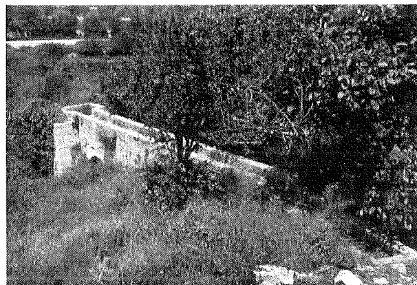
Fig. 3: Aqueduct and droptower of a watermill in Kritou Terra, Paphos.
